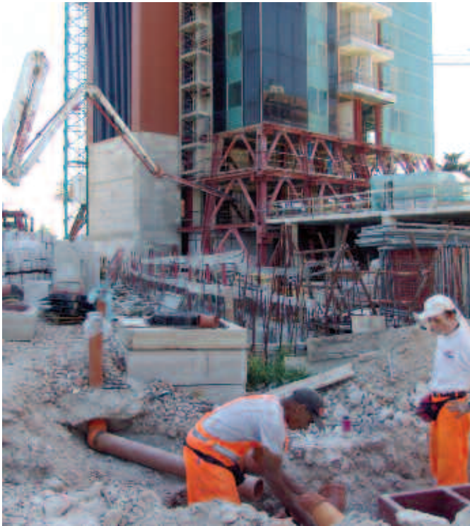
Cantiere edile a Bologna / Building site in Bologna
